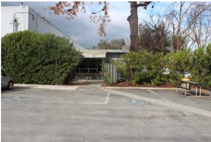
Figure 7: East façade covered patio area, looking west. Source: MIG, Inc., February 2016.
