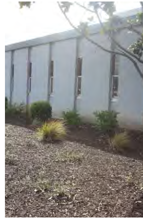
Figure 4: North façade plaster panels and obscured glass windows from Jefferson Drive, looking east. Source: MIG, Inc., February 2016.
