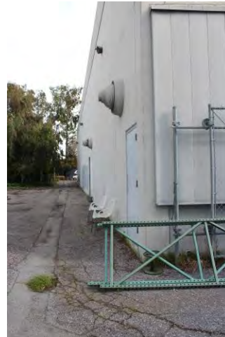
Figure 8: West façade with two exterior doors. Source: MIG, Inc., February 2016
