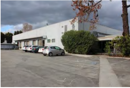
Figure 5: East façade showing loading garages and covered patio area, looking southwest. Source: MIG, Inc., February 2016.
