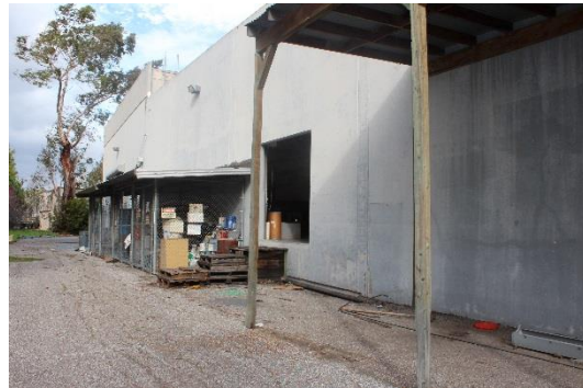
Photo 4: South façade with temporary awning structure, chain-link enclosure and loading door, looking northwest.
