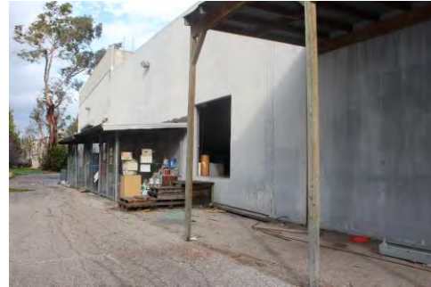
Figure 6: South façade with temporary awning structure, chain-link enclosure and loading door, looking northwest. Source: MIG, Inc., February 2016.
