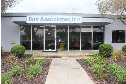
Photo 1: North main entrance from Jefferson Drive, looking south
