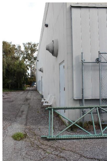
Photo 6: West façade with two exterior doors.
