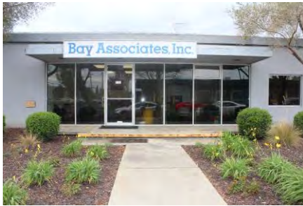
Figure 2: North main entrance from Jefferson Drive, looking south. Source: MIG, Inc., February 2016.
